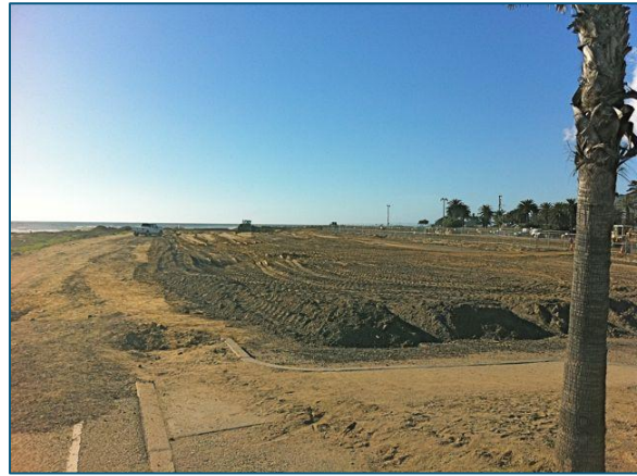
Removal of Parking Lot
