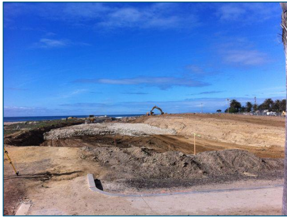
Excavation of Retreat Zone/Cobble Berm
