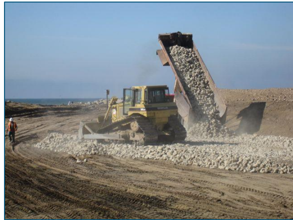
Importing of 6- to 18-inch Diameter Cobble
