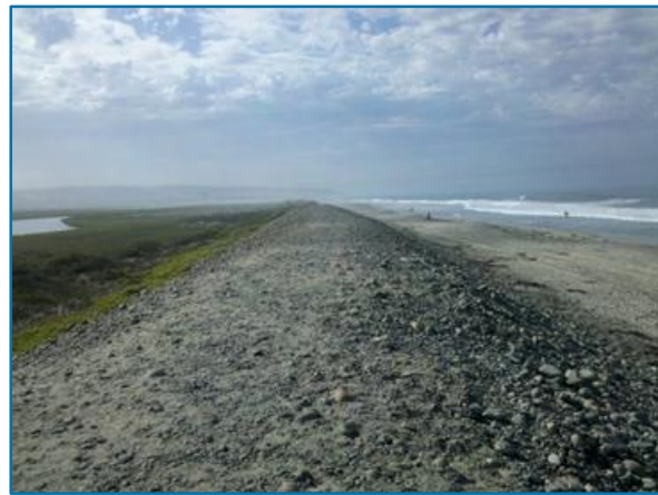
Figure 14: Crest Cobble Berm Looking South
