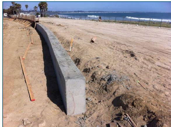
Construction of Parapet Wall
