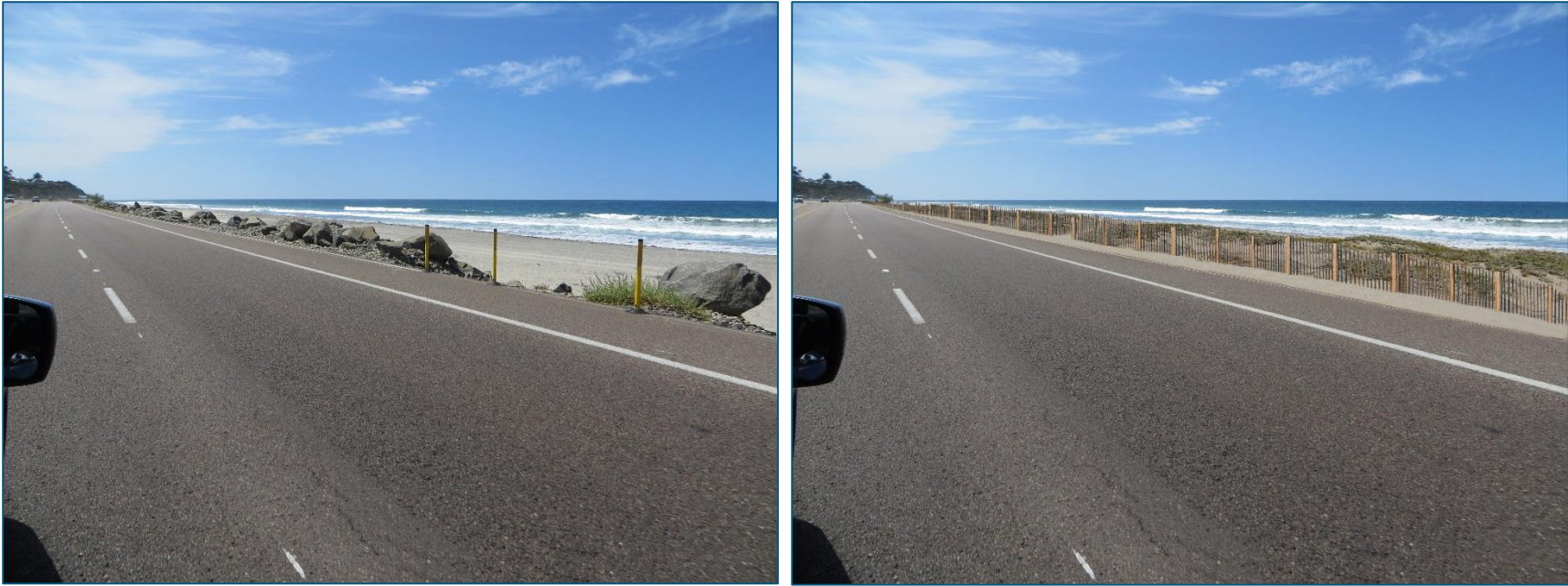
Figure 42: Photo Simulation of Sand Fence with Foot Trail and Lateral Beach Access Way View from HWY 101 southbound (#2 lane) (existing – left, proposed – right)
