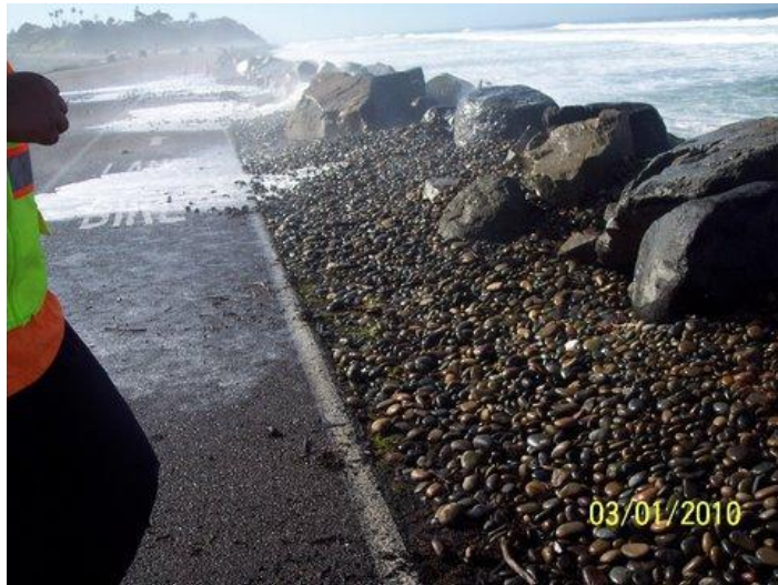
Flooding of HWY 101
