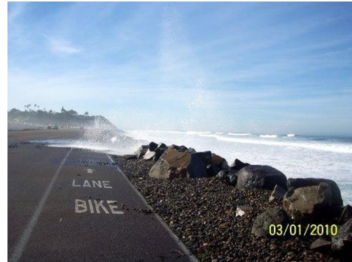
Flooding of HWY 101
