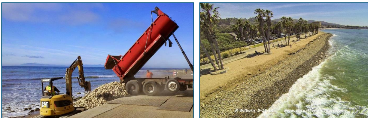
Figure 11: C Street Cobble Berm Construction in 2014 (Venturariver.org)
