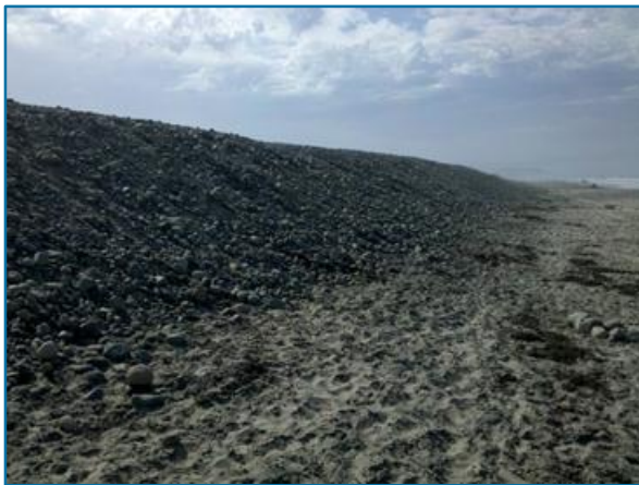
Figure 13: Cobble Berm in Imperial Beach
