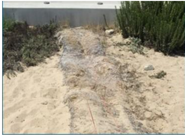
Sterile Rice Straw used to Stabilize the Sand while Vegetation Established
