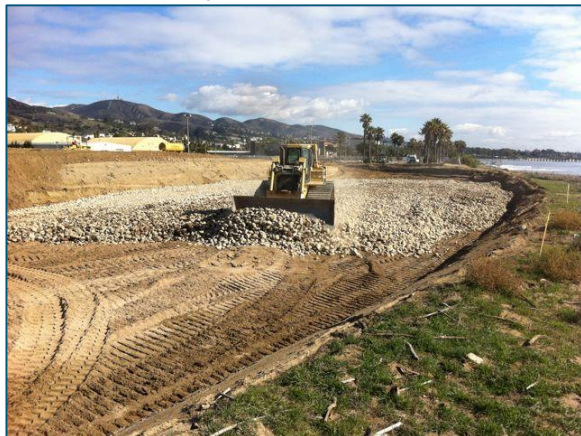
Construction of Cobble Berm
