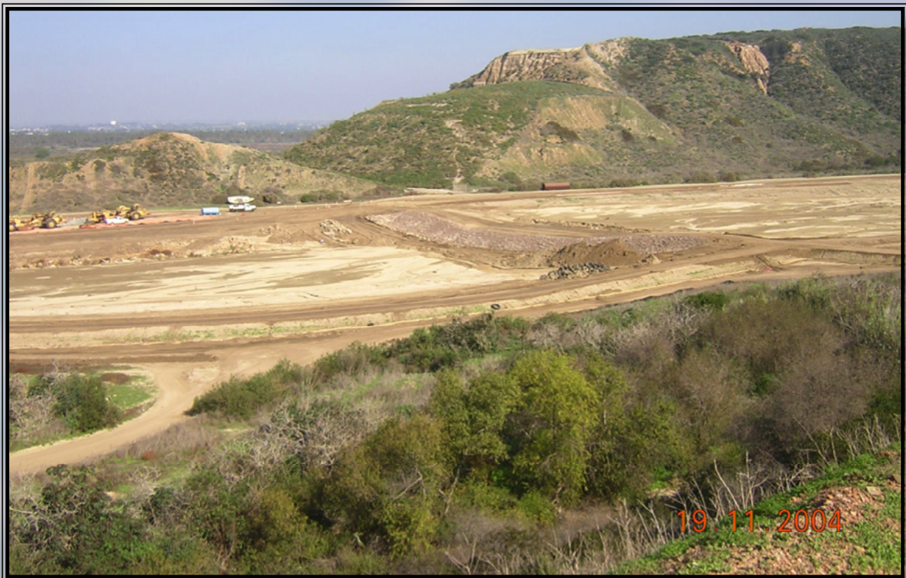
Goat Canyon before sediment basins had enough riprap to stabilize the berms; photo taken just after the Nov. 2004 deluge.
