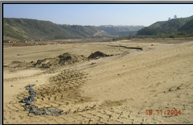
Goat Canyon before sediment basins had enough riprap to stabilize the berms; photo taken just after the Nov. 2004 deluge.
